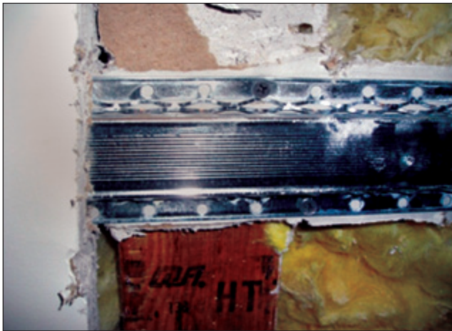
Figure 3. Double-screwed ceiling resilient channel (in original ceiling).
