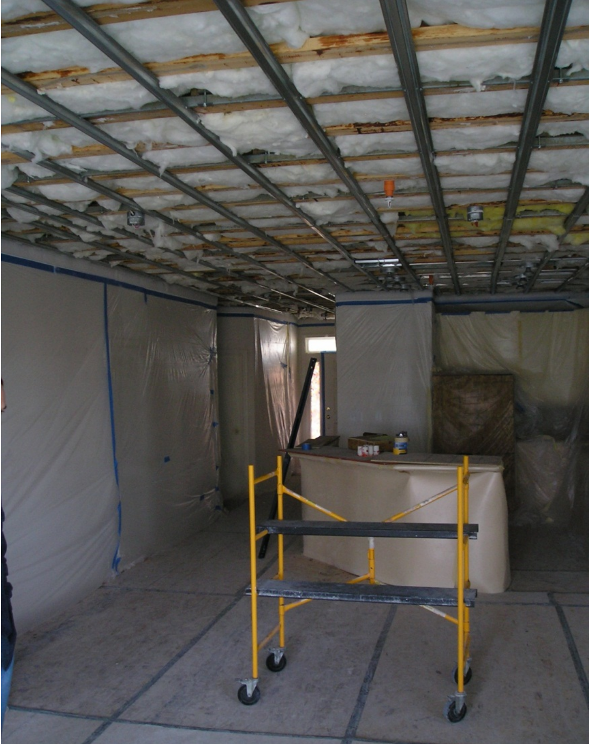
Fig. 8 – Existing ceiling demolition and spring isolated ceiling installation.
