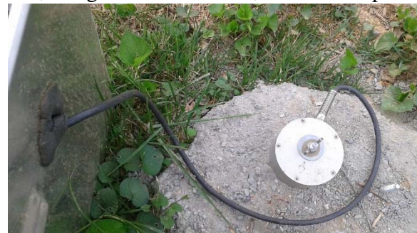
Figure 3 Accelerometer stud mounting in ground poured concrete
