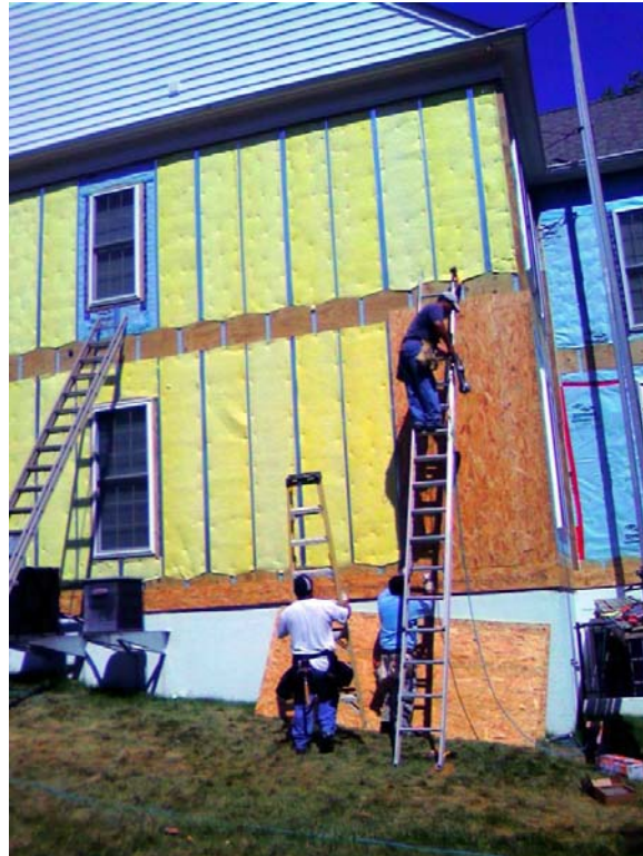
Figure 8: Construction of resilient channel option.
