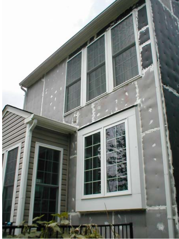
Figure 7: Construction of loaded vinyl option.
