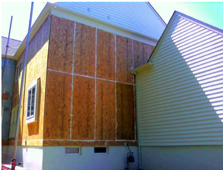
Figure 10: Resilient option showing final OSB and caulking.
